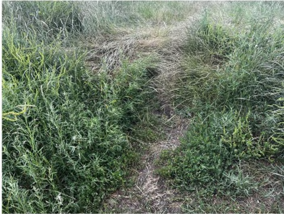
Sea wall at path to dock well vegetated and good condition
