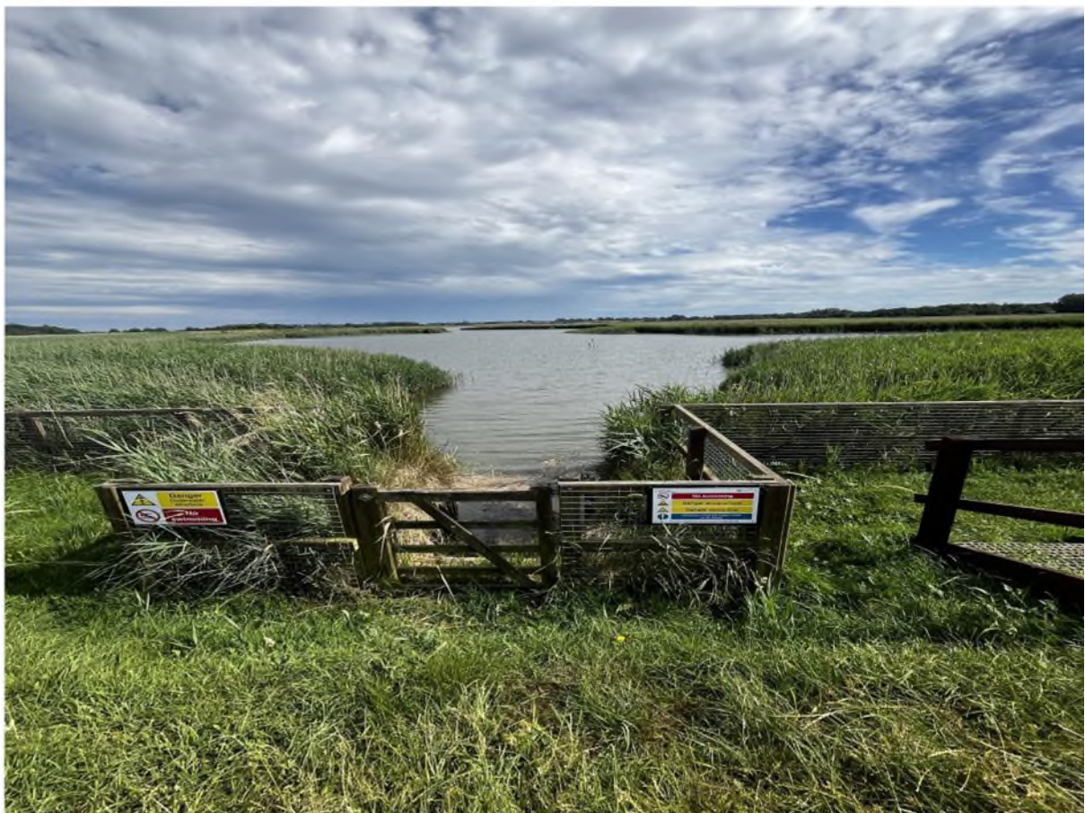
Sluice in good order
