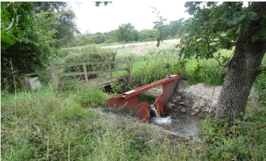
Fig. 1: Footbridge and V-notch weir at Valley Farm. Weirs such as this are often constructed on rivers and streams to enable the rate of flow to be measured.
