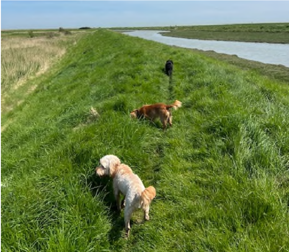
Photo 1 – Grid reference 52°04.381'N, 1°45.701'E. - Walls generally good condition
