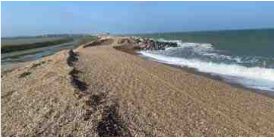
Looking north at pinch point.
