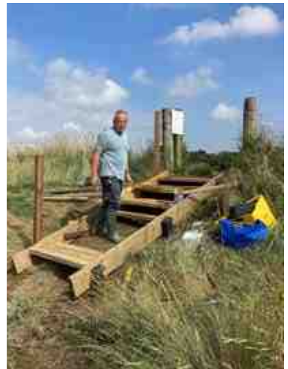
Volunteer James Walker in charge of step construction.
