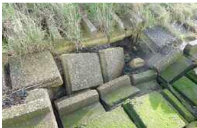
Damaged block revetments to be repaired.
