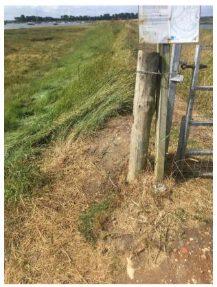
**Wall cracking:** On the wall footpath above Short Reach along the recently refurbished all from 455555 to 445560 in **Summer** there is significant surface cracking with fissures up to 10cm in width and indetermined depth, but at least 4cm. Whilst the clay path surface is 'crazed' there is no evidence of significant cracking in the winter months.
