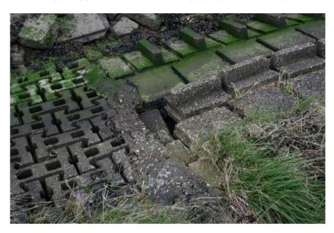
ii. Between the gate with steps to Dump Road at 458557 and Corporation Sluice the low protective wall ends. At this point two 'caves', identified in previous reports, remain, one now 3' wide v x3'6'' high, visible in photo below, and one 3' x2'high 15 yards to the west barely 2' below the top of the wall and is now undercutting beneath the footpath. Photo below
