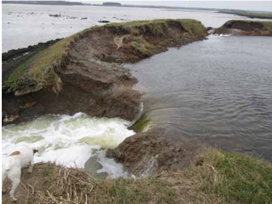
Figure 28. Two breaches in the river wall at Hazelwood Marshes created on 6 th December 2013; photograph taken 3 rd March 2014
