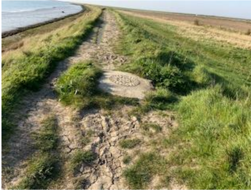
Photo 7 [manhole cover] [N52 05 14.659 E1 32 09 048]
