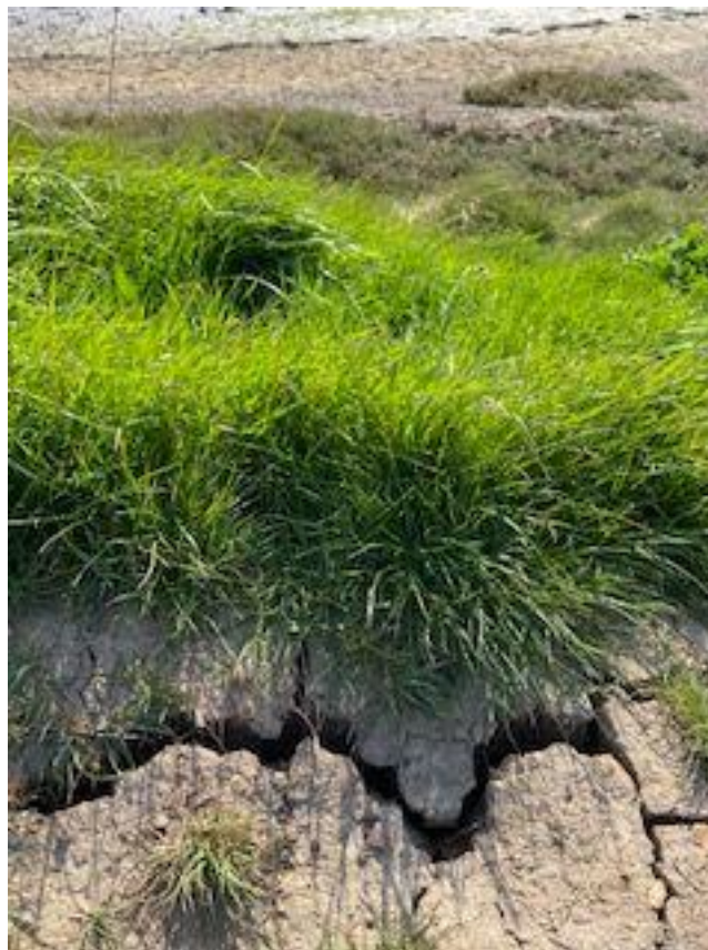
Photo 6 [cracked edge] [N52 05 18.19 E1 32 09.750]
