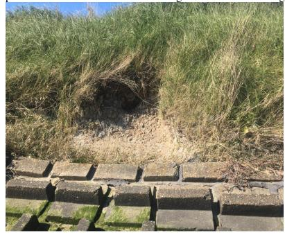
iii. start of undermining of older concrete protection at join with the new armorlok (new about 10 years ago) and old blocks collapsing at the top
