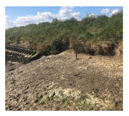
ii. large 'cave' (2 ft. high) in bank above the concrete protection has increased further making wall vulnerable to large waves.
