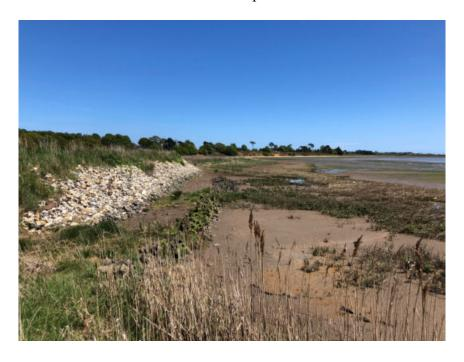
There are plans to raise the wall to 3.5m. However, the wall is in good shape, apart from the top slopes to the back. There is good vegetation and the wall profile is fine.
