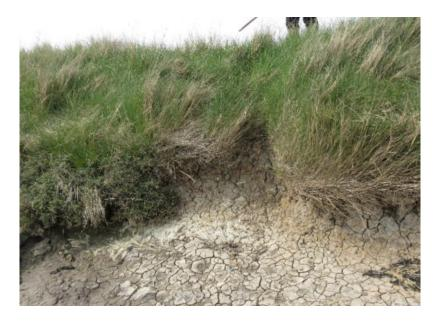
iii. West of sluice outlet, two patches of concrete blocks caving in with erosion of clay from behind (photo) one with hollow behind TM 458557
