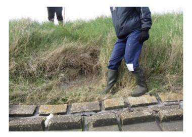
ii. New erosion of clay bank 6-8ft to east of armorlok protection TM 459557
