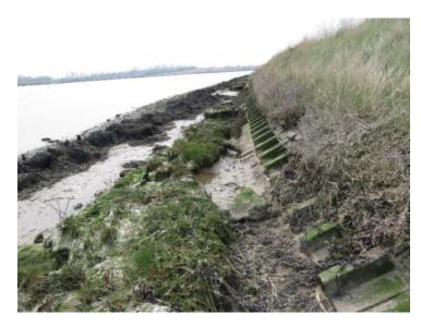
v. Saltings pilot project - in most cases (5 sites) the hazel bundles behind the tensar fencing plastic has disappeared. Not clear how much protection the tensar offers - needs monitoring by AOEP.
