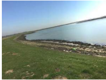
Last stretch towards Chantry Point – pathways in poorer condition than elsewhere in this part of FC4, some mud and seaweed covering up generally sound revetments, no significant changes.
