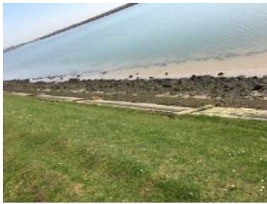
Last stretch towards Chantry Point – pathways in poorer condition than elsewhere in this part of FC4, some mud and seaweed covering up generally sound revetments, no significant changes.
