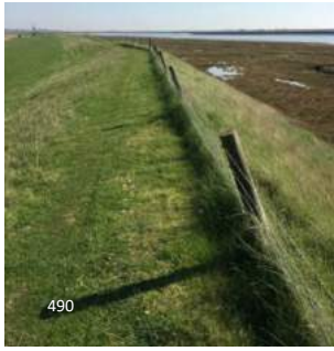
At 408 473, path towards the pumping station – fence posts have started to lean in again after recent repairs; saltings channel and some undercutting visible; general view.
