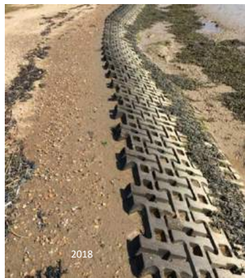
River wall revetment around 411 475, last year and this. At the top of the line of linked defence slabs the mud/shingle is washing away, leaving the top of the revetment exposed.
