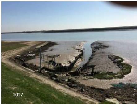
At 408 473, path towards the pumping station – fence posts have started to lean in again after recent repairs; saltings channel and some undercutting visible; general view.
