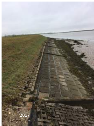
River wall revetment around 411 475, last year and this. At the top of the line of linked defence slabs the mud/shingle is washing away, leaving the top of the revetment exposed.
