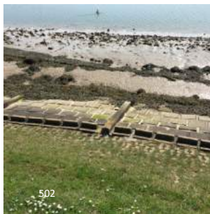
Revetment slabs buckling slightly at 411 476; worn and damaged pathway at this point; generally sound revetments and more evidence that (? sheep) a small track is being created at the outer foot of the wall at around 412 477.
