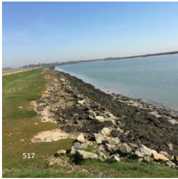
Coming towards Chantry Point – rock defences and bare patches in the pathway and outward wall at 412 477; more recently placed rock defences at 412 478
