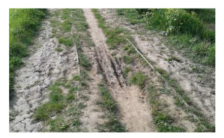
**Saltings:** Brick Dock 448562 to 449565. Most of the tensar fencing material has come away from the piles, clearly not up to withstanding the strong westerly fetch waves and movement at the bottom prevents accumulation of silt (reported to AOEP saltings group).
