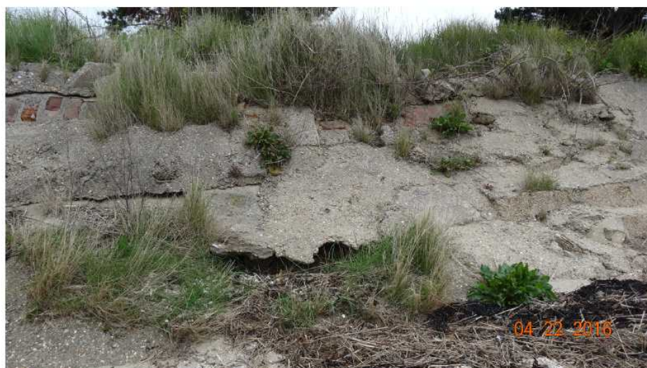
Erosion to wall at Roundhill
