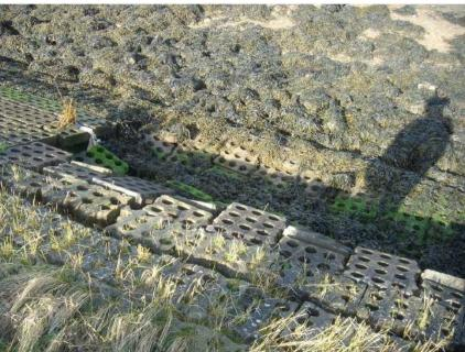
5640-4320 evidence of saltings erosion in the bays. We noted one occasion where a channel has formed between a good stretch of saltings and the wall. Is this a risk? ie that the benefit of saltings can be lessened by such a channel?
