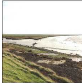
River wall at final bend and saltings general view at Chantry Point, 415 484 – path is worn but better grassed than last year, no visible change to saltings or river wall/slopes.
