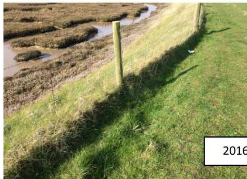
The path at 400473, in 2015 and 2016 – continued slumping by posts, and some evidence of slippage on wall facing river, but not worse than last year.
