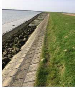
Boulder and shingle defences at 412478, revetment and damage (already grassed over) to river wall slope above at same place; lumpy landward slope well grassed over further along the pathway towards Chantry Point at 413479.
