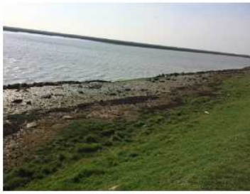
Boulder and shingle defences at 412478, revetment and damage (already grassed over) to river wall slope above at same place; lumpy landward slope well grassed over further along the pathway towards Chantry Point at 413479.
