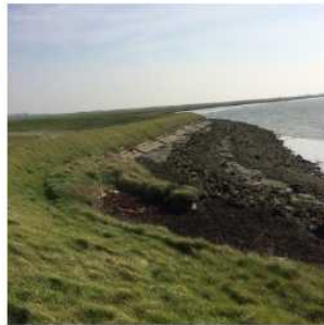
Pathway at 414483 / 415484 – very lumpy and uneven, some possible damage/slippage on river wall side
