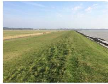
Boulder and shingle defences at 412478, revetment and damage (already grassed over) to river wall slope above at same place; lumpy landward slope well grassed over further along the pathway towards Chantry Point at 413479.
