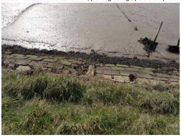
5. 393 508/7 Slight buckling of revetements and plant growth.
