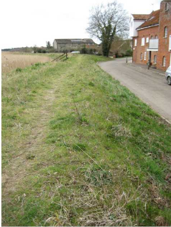
1 st 100 mtrs by Mill in reasonable condition
