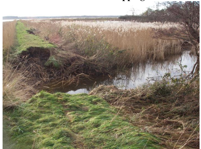
10 main Breach end of East wall close to sluice
