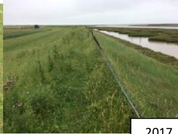
The path at 406 473, 2015-2017 – continued stumping by posts, and some evidence of slippage on wall facing river; no significant deterioration though.
