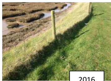
The path at 406 473, 2015-2017 – continued stumping by posts, and some evidence of slippage on wall facing river; no significant deterioration though.
