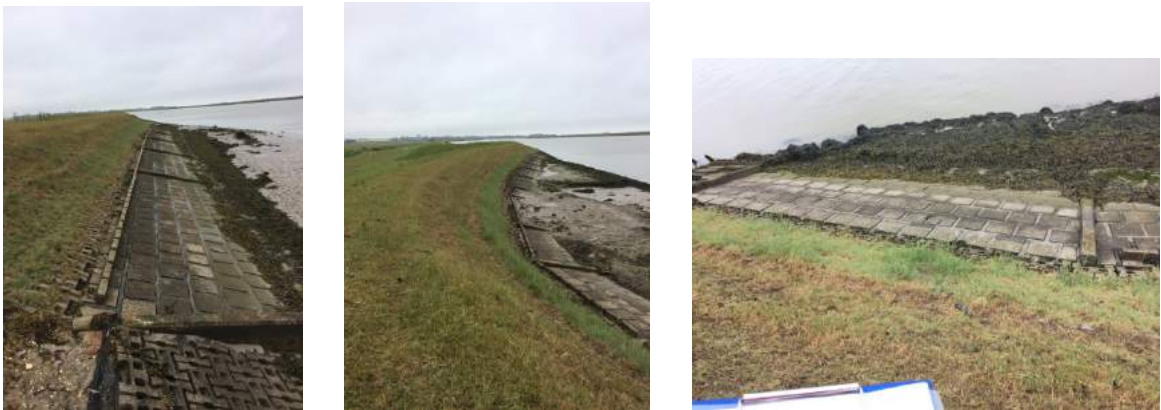
River wall revetment from 411 476 towards 412 477. Reasonable condition along this section.
