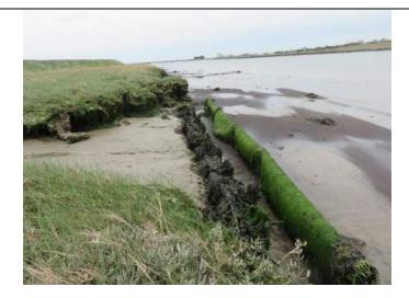
5. Brick Dock. TM 449564 Further failure of the pilot project tensar stretch, probably reflecting inability to cope with rolling waves resulting from long western fetch.
