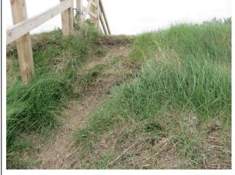
**4. Brick Dock surrounding wall.** This was fully repaired some three years ago. In a few places the armour is beginning to dip as the earth behind is washed out. There is no substantial deterioration at present but these slight slumped parts will need to be monitored carefully over the next few years and could be dealt with when Phase 2 of the Aldeburgh Marsh project is done. TM448563
